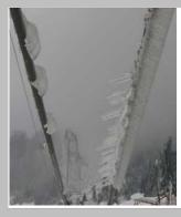
Significant reduction, in order of millions of €, of infrastructural reconstructions after catastrophic events due to extensive icing on overhead power lines. Such event last occurred in the beginning of February 2014, when a considerable number of transmission lines collapsed under the weight of accumulated ice glaze. The damage of this single event was estimated at 8.5 million €.
