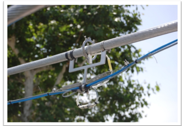
Fig. 4. Digital temperature sensor on the surface of a conductor loop connected to a communication data bus.
